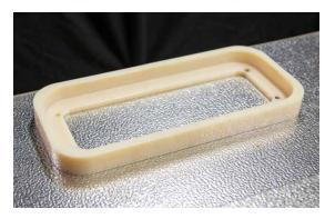
2. Drill  $\frac{1}{4}$ " starter hole at edge of template or plunge Roto-Zip tool into sheet metal surface near edge. Trace outline of template with tool, cutting out installation hole for 1826 unit.
