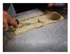
Once 1826 body fits flush into wall, proceed with install of wiring and other components to finish. Secure 1826 to wall skin using 4 screws.
