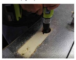
8. Use plunging router (not shown) to cut away rectangle of foam to correct depth and skip to step 10, or manually use hole saw to make starter cuts prior to step 9.
