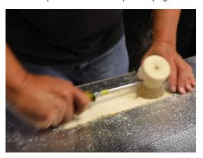
7. Using hole now available from hole saw cut, continue hole sawing until contact with opposite side sheet metal, then break out last plug of Styrofoam.
